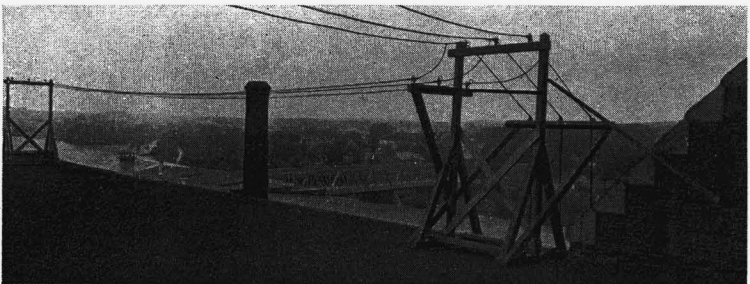
FIG. 19. SUBSTANTIAL WOODEN ROOF STRUCTURES.
